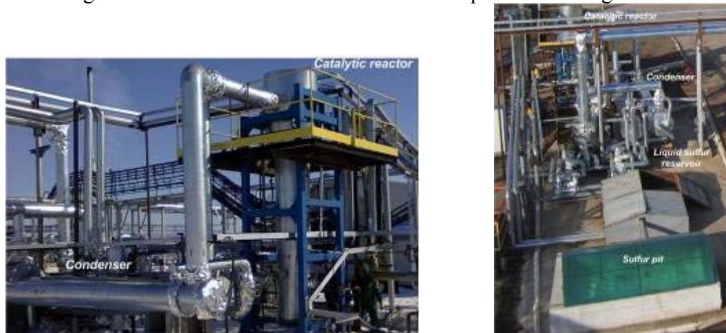
Figure 2: Industrial installation for direct selective oxidation of hydrogen sulphide
